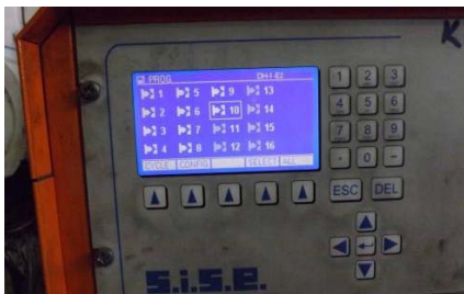
Fig 2 10. injection nozzles activated.
